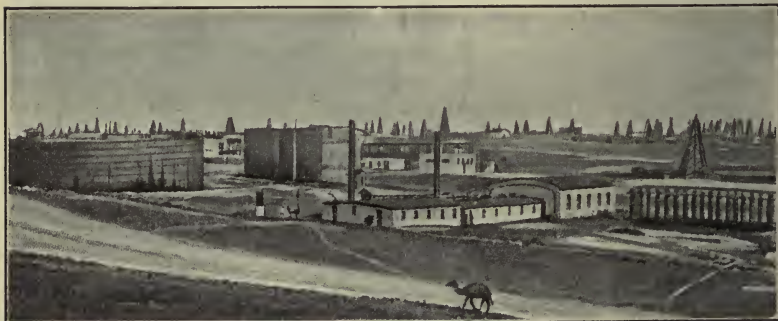
Fig. 288. — Oil wells and tanks, Russia.
