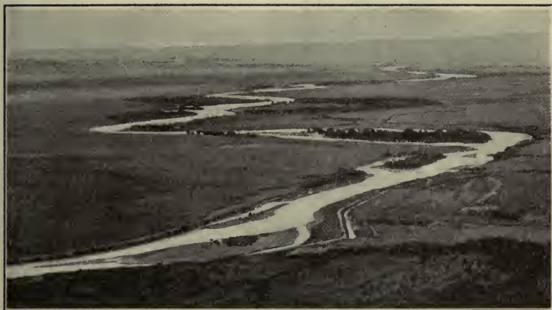
Fig. 94. — Bighorn River in the plains, Wyoming. Irrigation canal on right bank.
