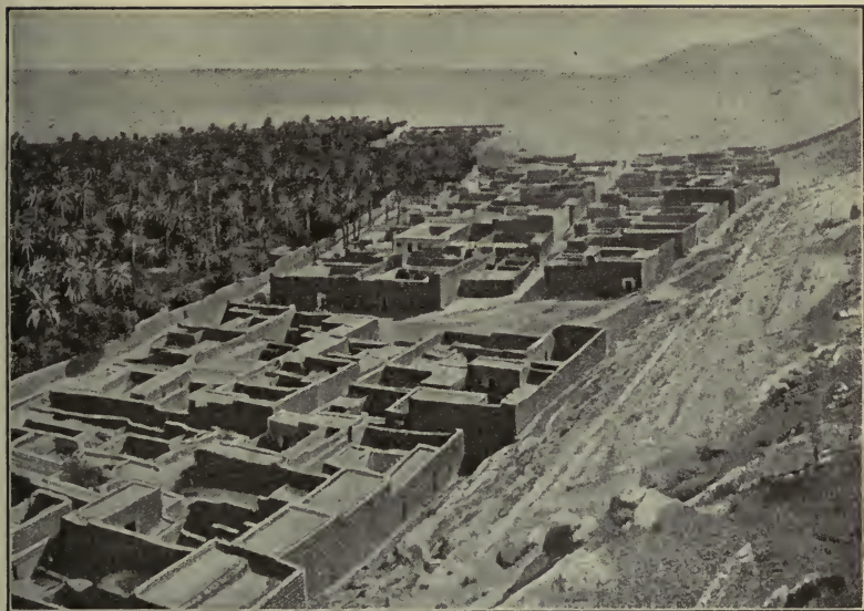
Fig. 206. — Date palm oasis, Sahara. Note flat-roofed houses.
