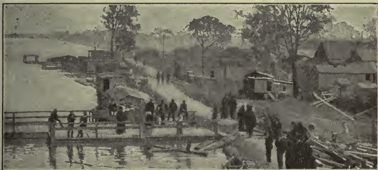
Fig. 100. — A Mississippi levee, Greenville. High water above the level of the town.
