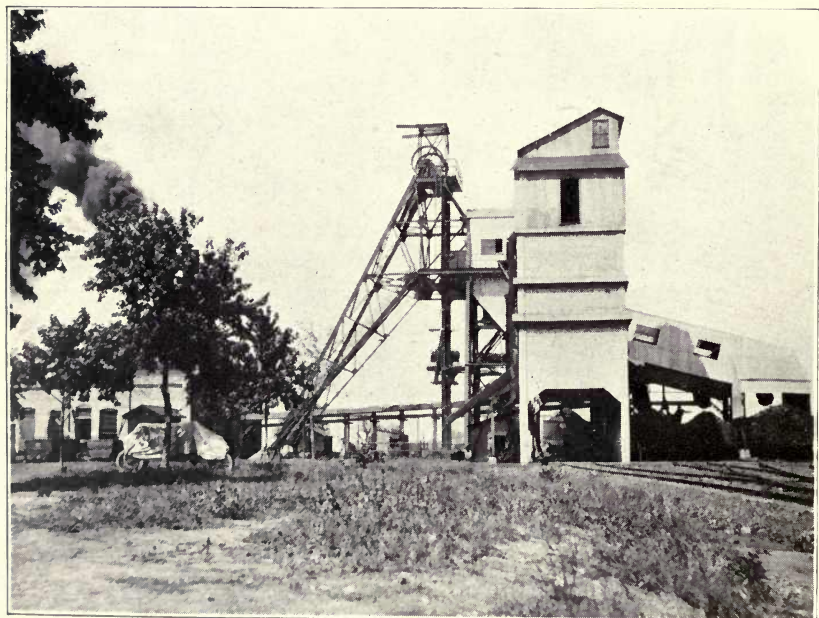
FIG. 2. A MODERN STEEL TIPPLE WITH CONCRETE RESCREENER.
