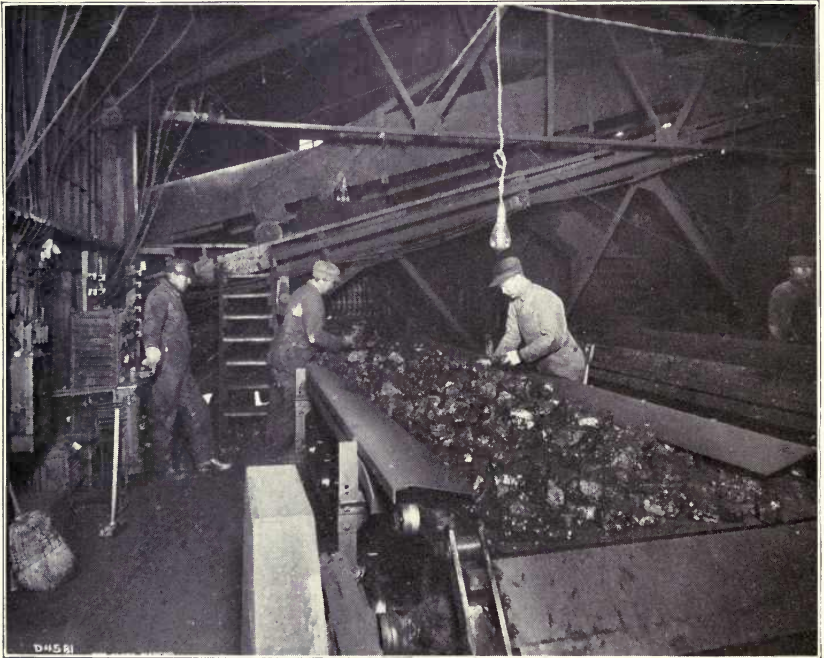
FIG. 19. OPERATION OF A PICKING TABLE.
