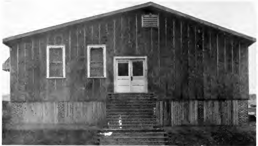
FRONT VIEW — ADMINISTRATION BUILDING — N.C. COLLEGE FOR NEGROES
