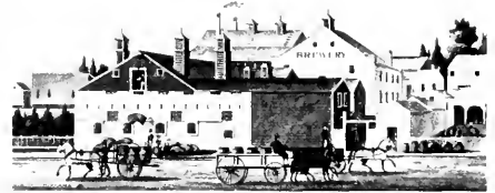
The Vassar Street Brewery, Bridge Street Front, from a drawing made by Henry Whinfield in 1837.
