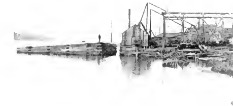
Bridge Caisson, Ready to float to Position, 1877.
