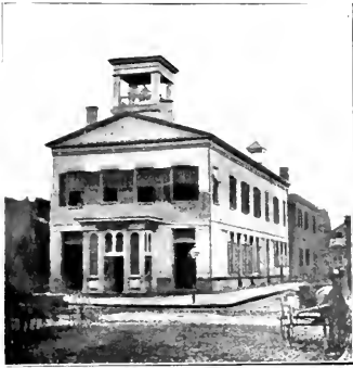
The Village Hall, now the City Hall. Photographed in 1880, when the rear building was erected.
