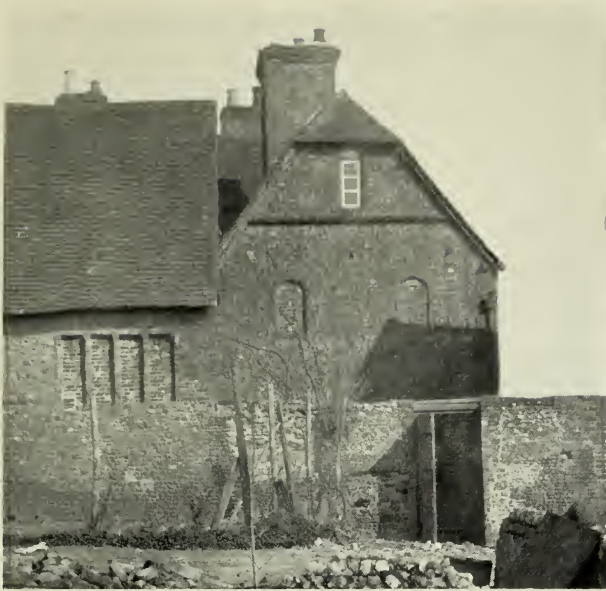
West side showing the blocked windows
