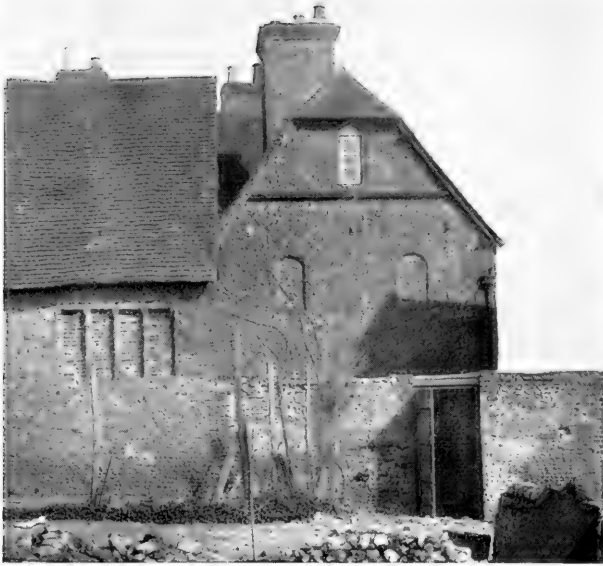
West side showing the blocked windows
