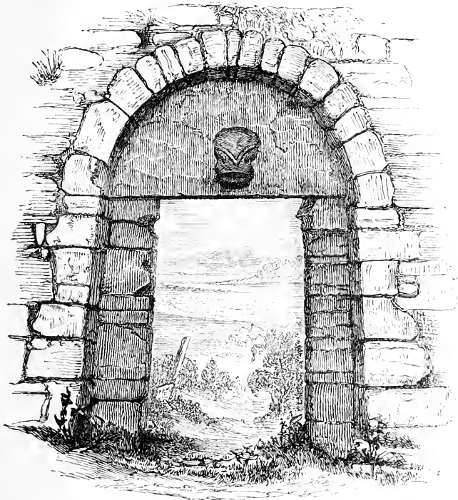
FIG. 87.—DOORWAY OF KILMALKEDAR (INTERIOR).
