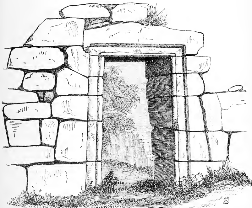
FIG. 78.—DOORWAY OF TEMPLE MARTIN, KERRY.
