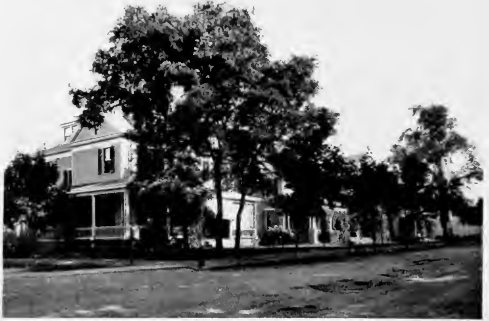
South College Street. Home of Dr. Morris W. Prince on the Corner
