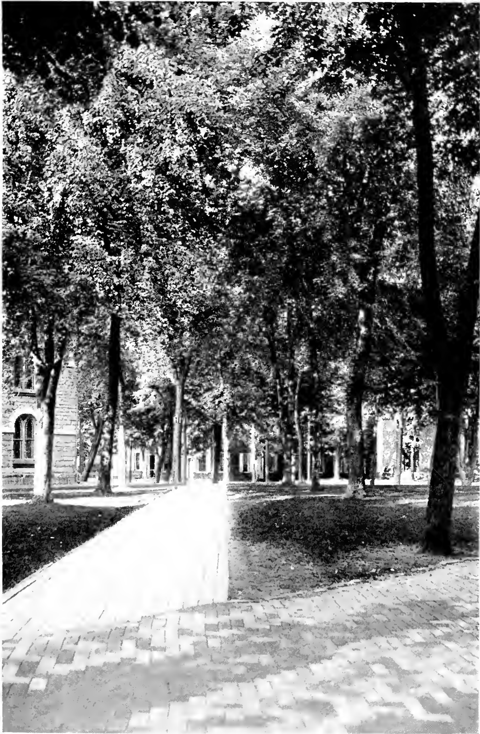
Public Square and Corner of First Presbyterian Church
