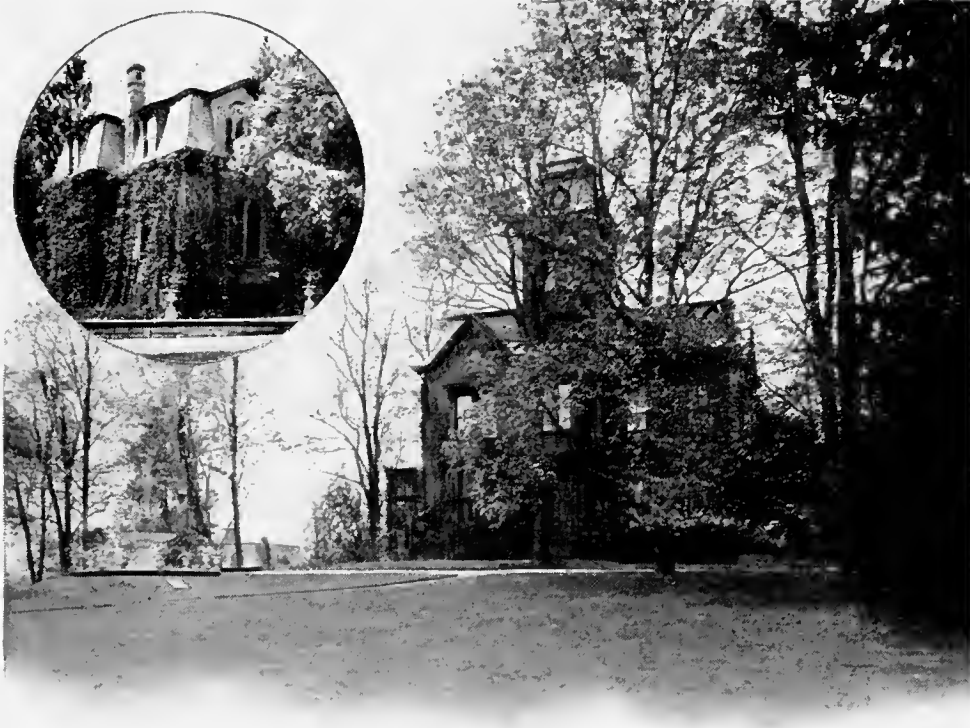
"Cottage Hill" and Vine-clad Office of F. C. Bosler, Esq.
