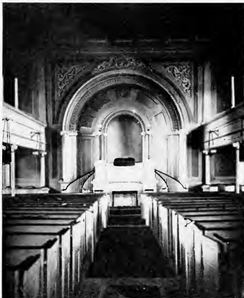
Interior of First Presbyterian Church. From 1827 to 1876
