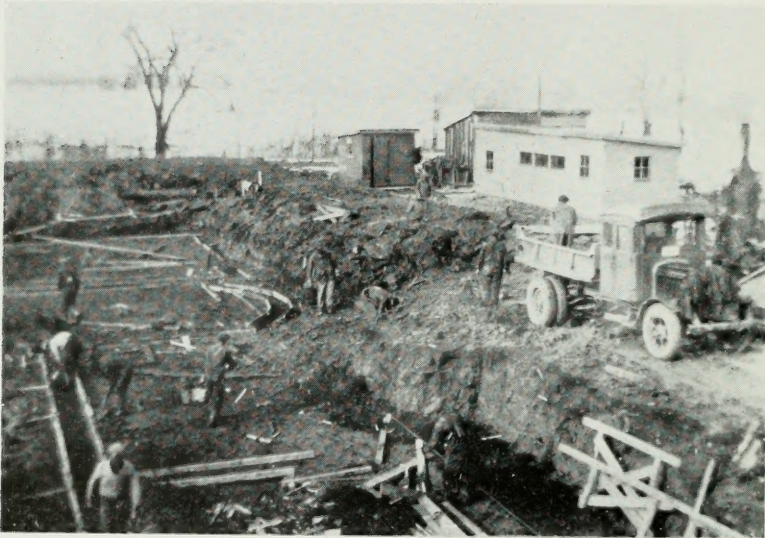
Foundation-work on new Lower School Building.
