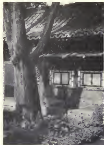
House in Peking. 194
