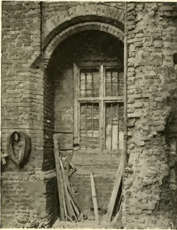
(a) ARCH UNDER CHIMNEY-STACK
