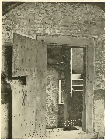
(c) SECOND FLOOR, STAIRCASE
