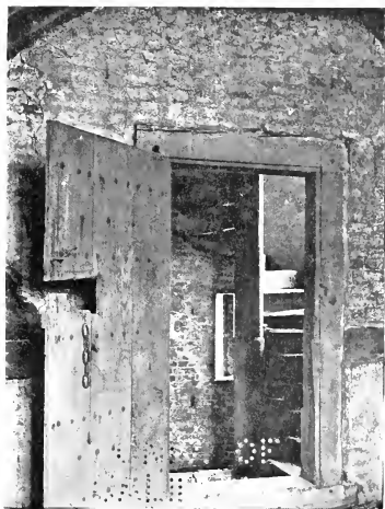
(c) SECOND FLOOR, STAIRCASE
