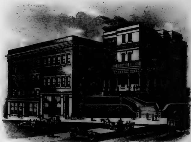
BUILDINGS FOR OFFICE PURPOSES 10TH & OAK STREETS
