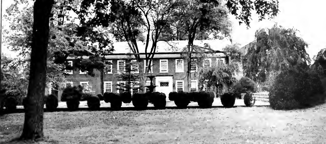
Arts and Science Building
