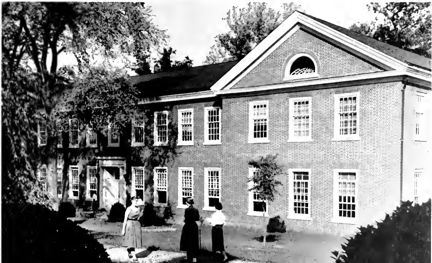
Arts and Science Building
