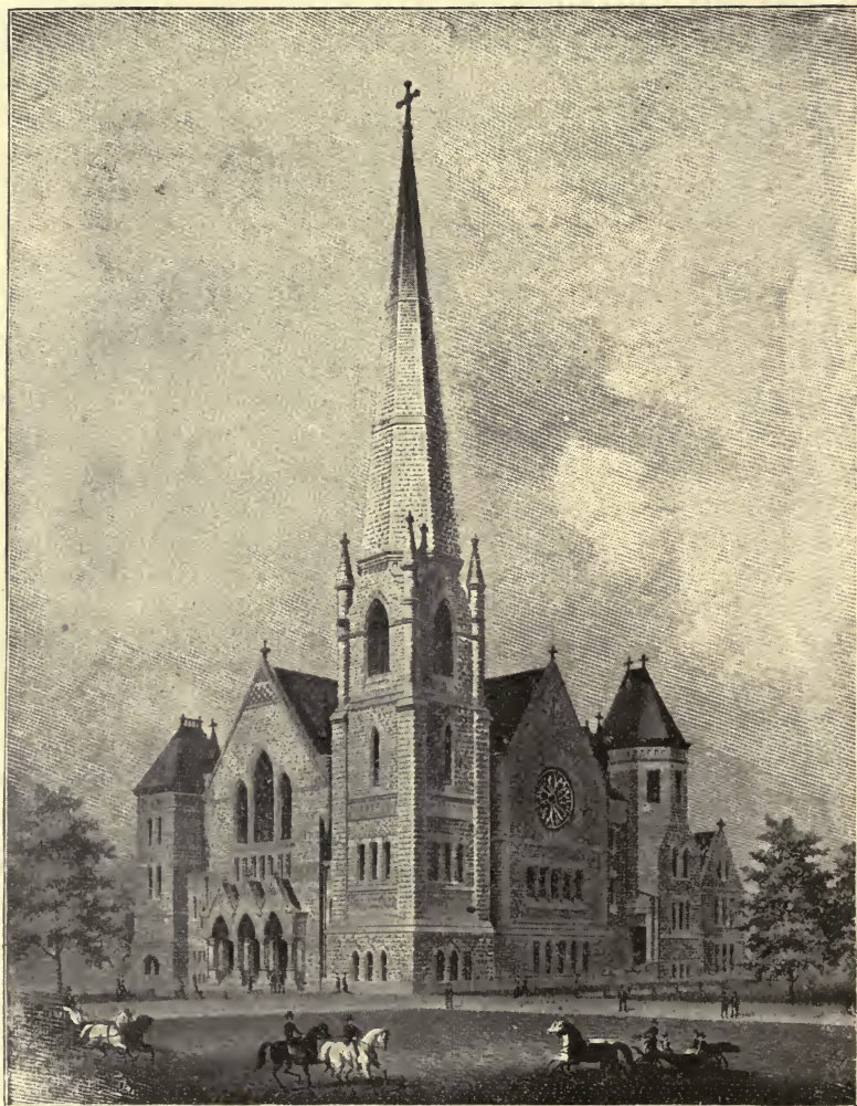
TRINITY METHODIST EPISCOPAL CHURCH, DENVER, COLORADO.
