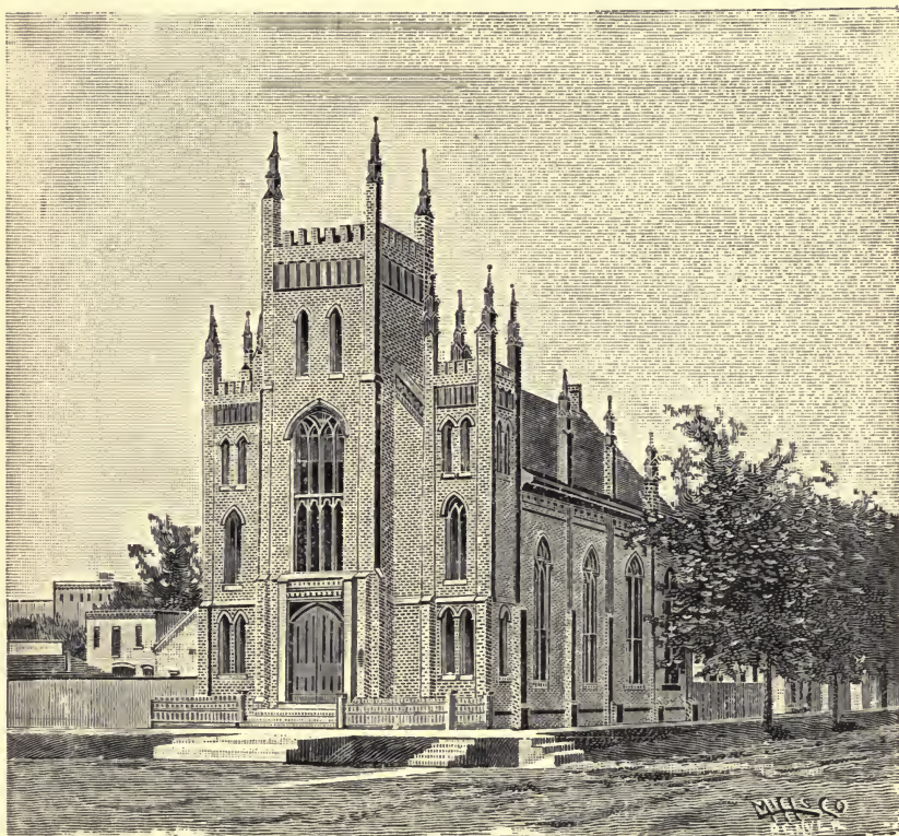
LAWRENCE STREET METHODIST EPISCOPAL CHURCH, CORNER OF FOURTEENTH AND LAWRENCE STREETS.
