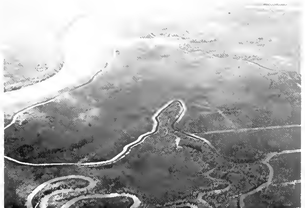
Figure 46. The extent of diking by agricultural interests along the western bank of the lower Apalachicola River.
