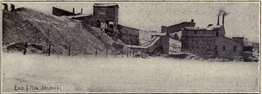
FIG. 132.—Zinc mine and mill of the Northern Ore Company, Edwards, New York.
