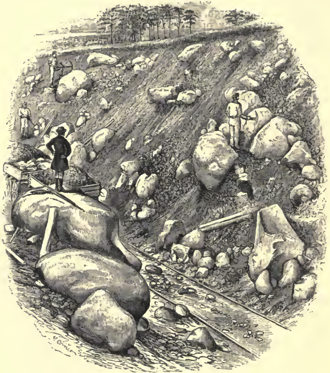
Cutting through Boulder-Clay, Linlithgowshire.
