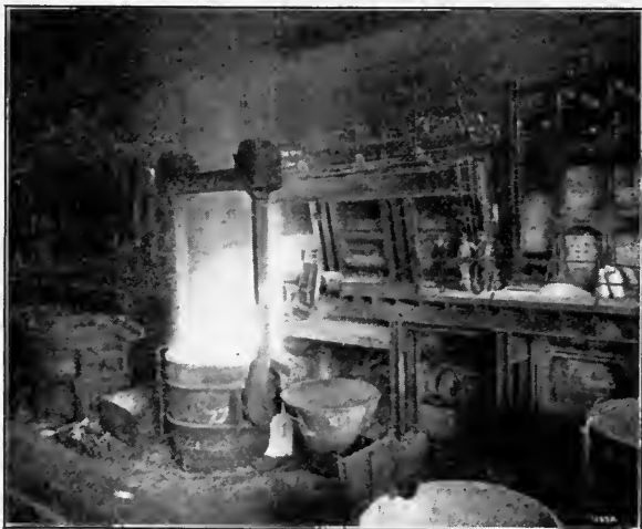
Tapping an Open Hearth Furnace
