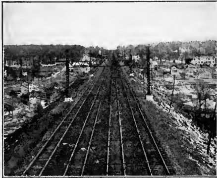
Electrification on the New York, New Haven and Hartford Railroad. Overhead Transmission.
