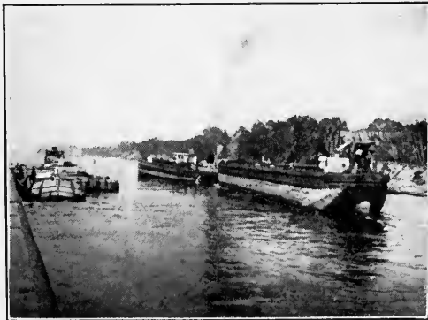
Modern Barge on the New York Barge Canal State Engineer and Surveyor's Department
