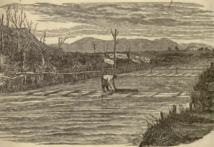
"FLY CATCHING," OR COLLECTING FLOAT GOLD.
