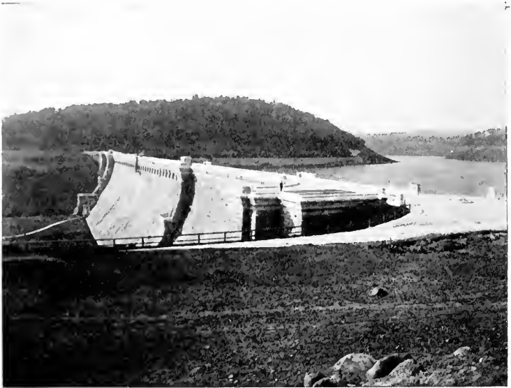
A PUBLIC ENTERPRISE N. Y. City water supply dam at Croton, N. Y.
