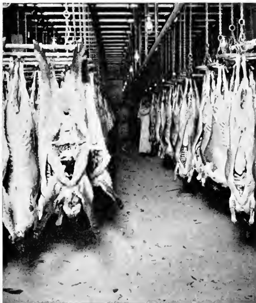
Cold storage plant
