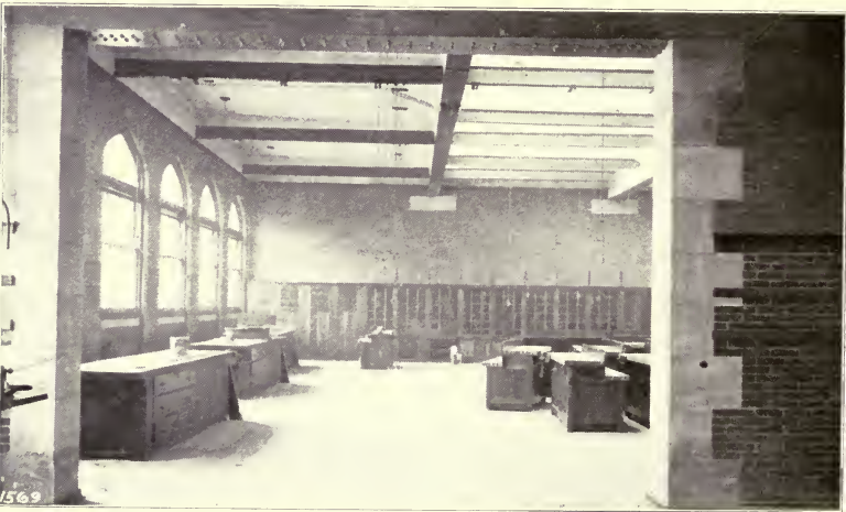
Fig. 67. Pattern Shop Chicago Manual Training School, showing Distribution of Light from Saw-Tooth Roof.
