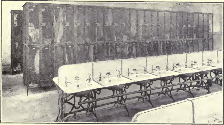
Fig. 18. Lockers and Wash Room.
