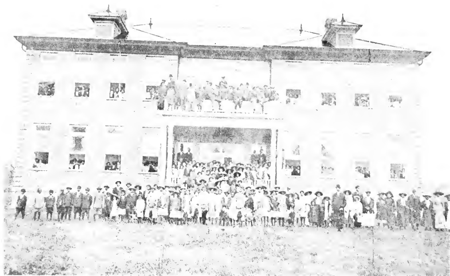
OLD ADMINISTRATION BUILDING
