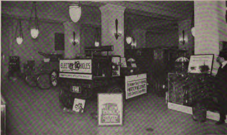
Photograph by The New York Edison Company
