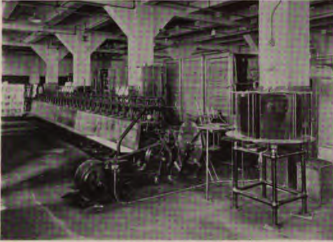
Photograph by The New York Edison Company
