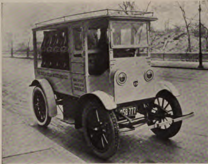
Photograph by The New York Edison Company
