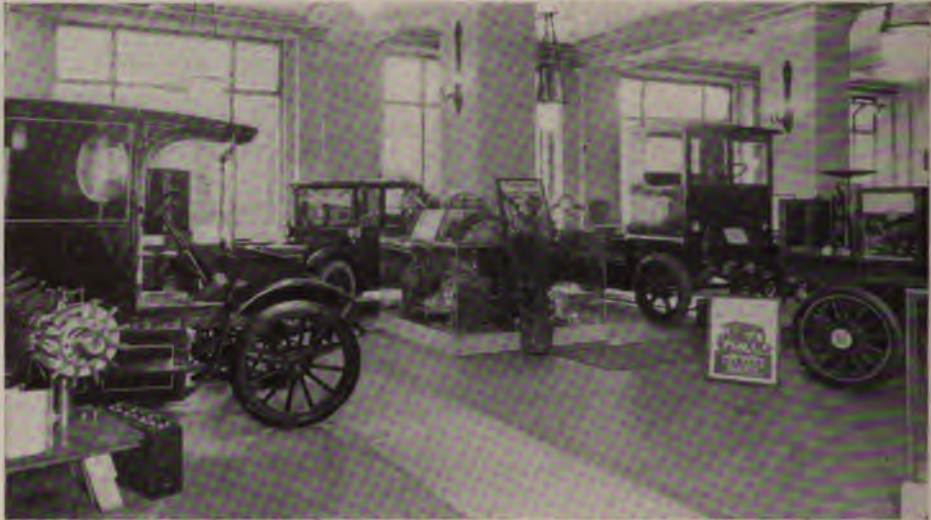
Photograph by The New York Edison Company
