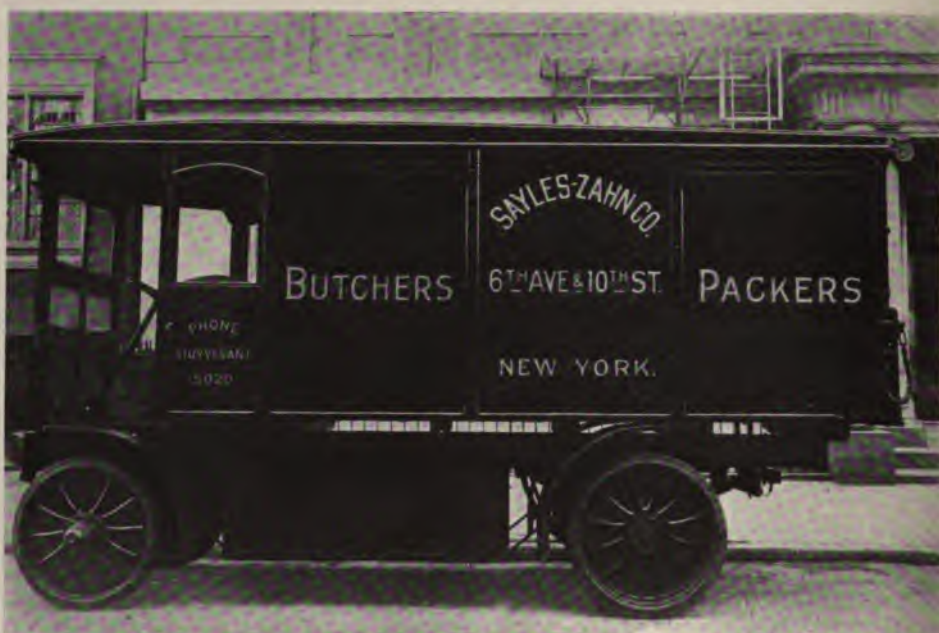
Photograph by The New York Edison Company
