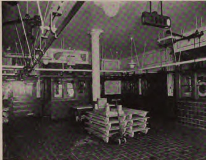
Photograph by The New York Edison Company
