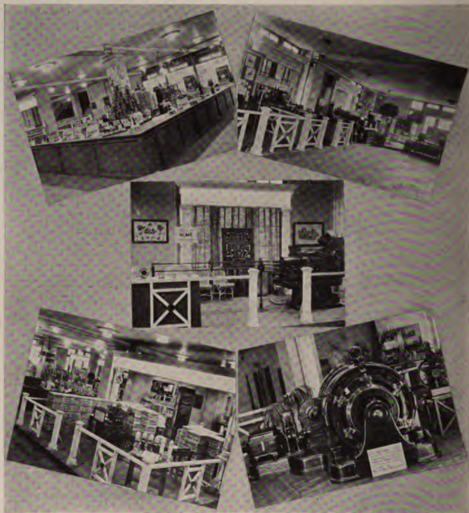
Photograph by The New York Edison Company
