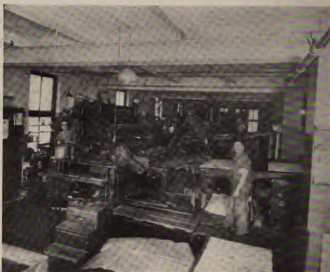
Photograph by The New York Edison Company
