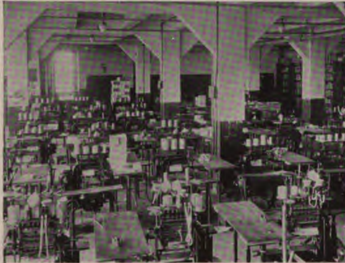
Photograph by The New York Edison Company
