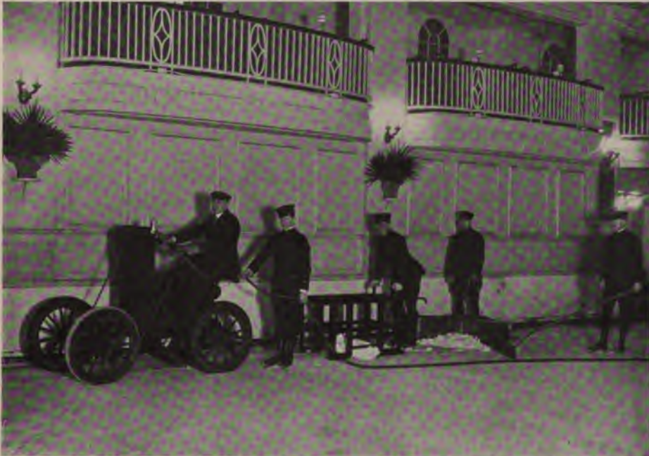
Photograph by The New York Edison Company
