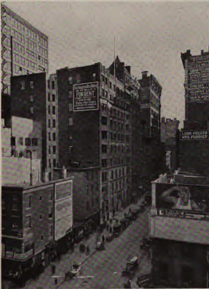
Photograph by The New York Edison Company
