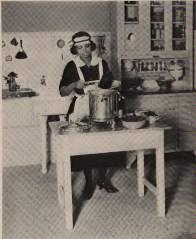
Photograph by The New York Edison Company
