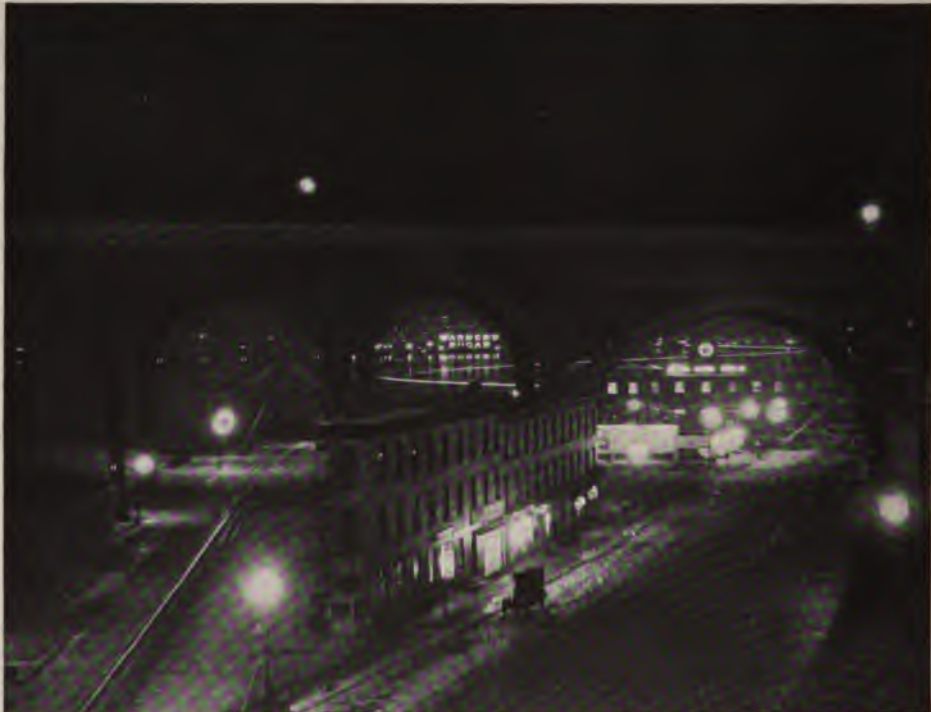
Photograph by The New York Edison Company
