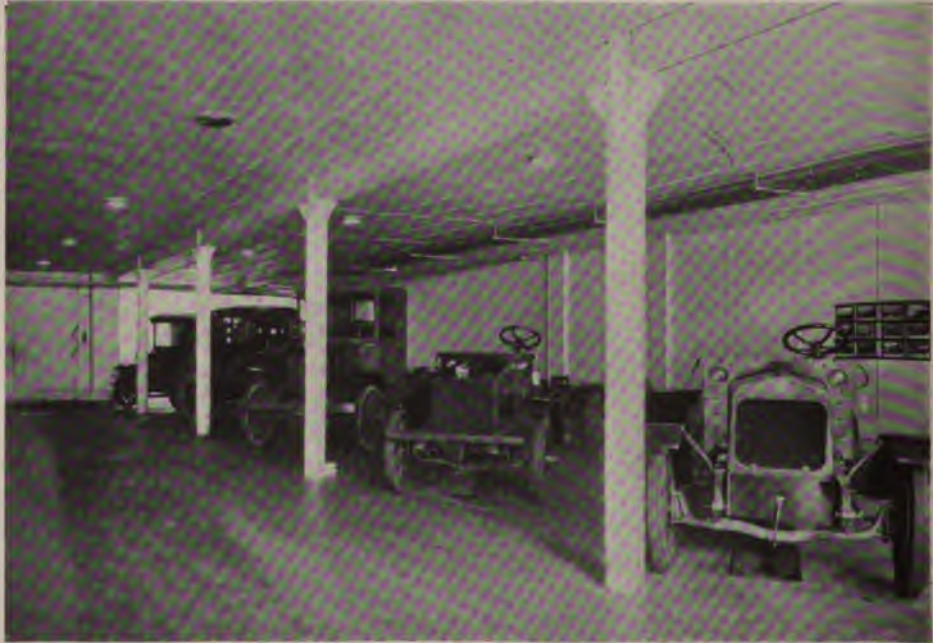
Photograph by The New York Edison Company
