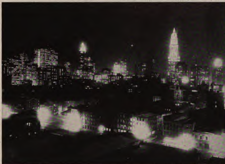
Photograph by The New York Edison Company
