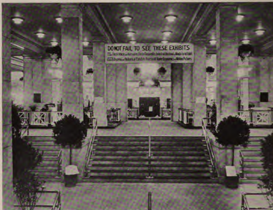
Photograph by The New York Edison Company
