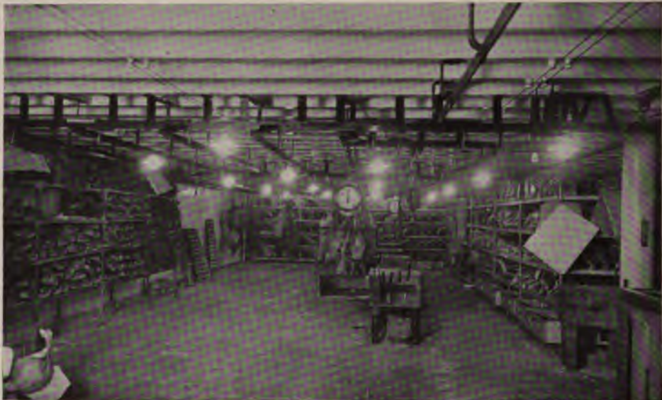
Photograph by The New York Edison Company
