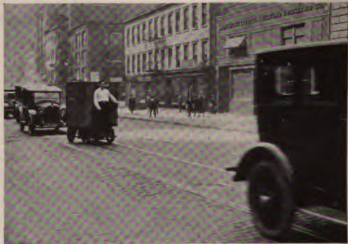
Photograph by The New York Edison Company One of the Efficient Little Electric Mail Trucks Making a Journey Down Fourth Avenue. An Electric Industrial Truck of This Kind is Easily Operated in Streets Where the Traffic is Congested
