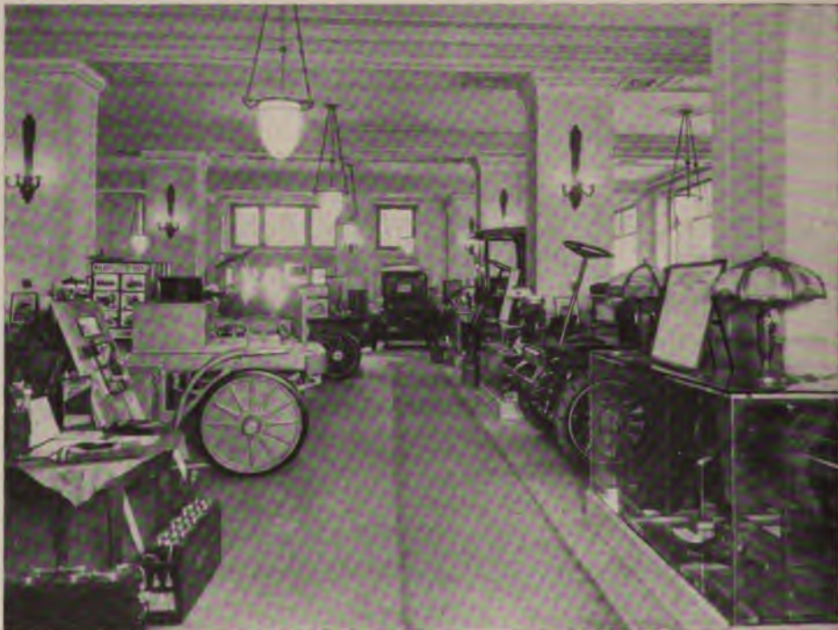
Photograph by The New York Edison Company
