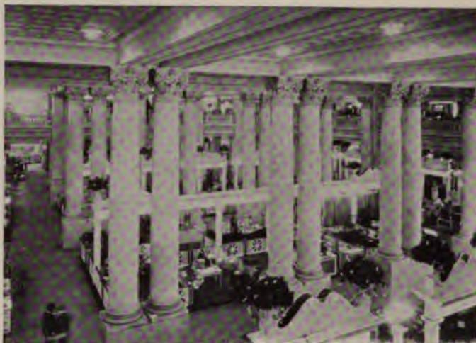
Photograph by The New York Edison Company Looking Down on the Main Floor from the Mezzanine
