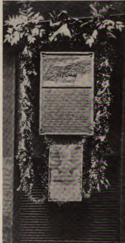
Photograph by The New York Edison Company
