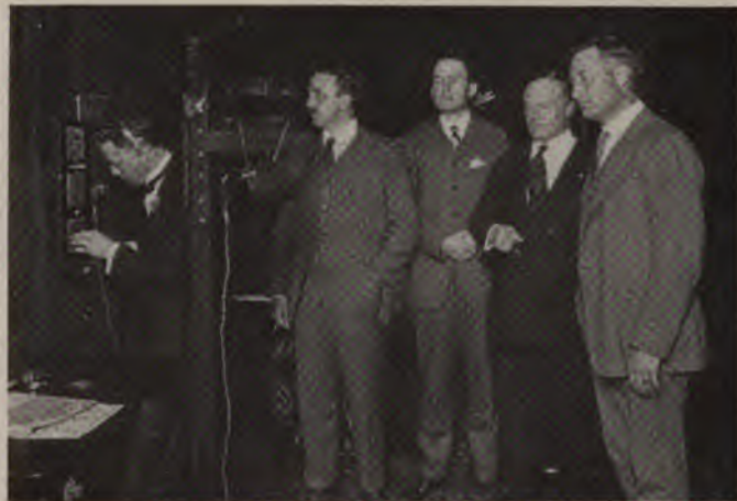
Photograph by The New York Edison Company
