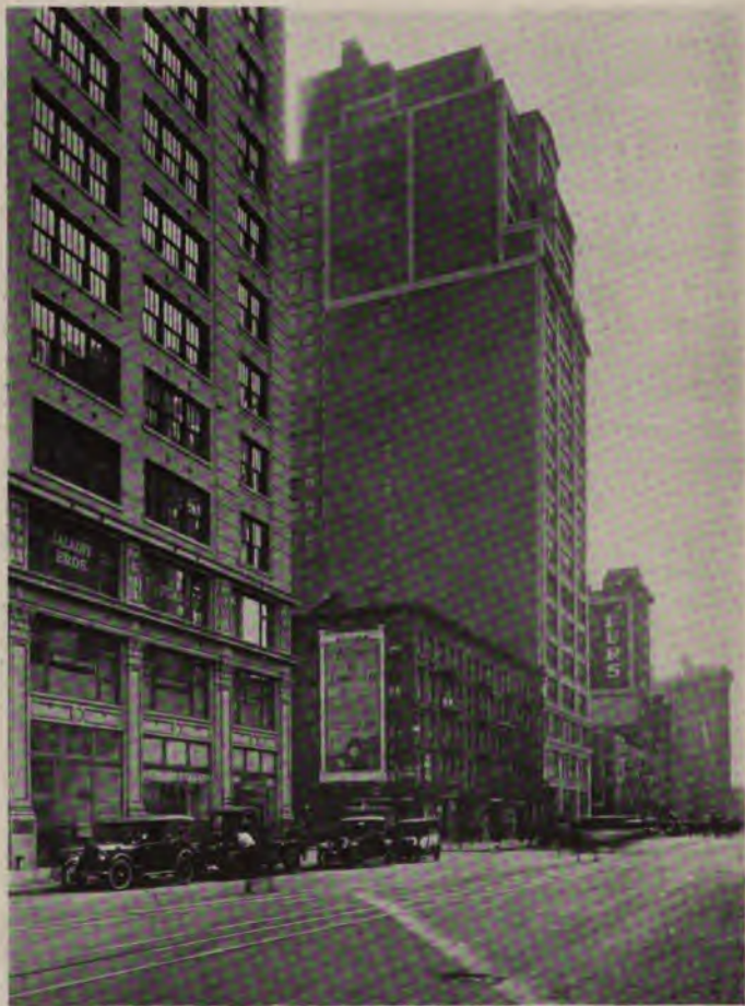
Photograph by The New York Edison Company Seventh Avenue is the Main Artery of New York's Fur District, and New Loft Buildings Are Rapidly Replacing the Five-and-Six-Story Structures of an Earlier Day
