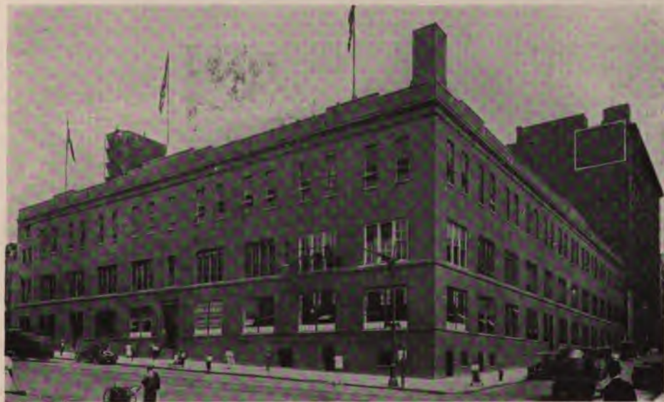
Photograph by The New York Edison Company
