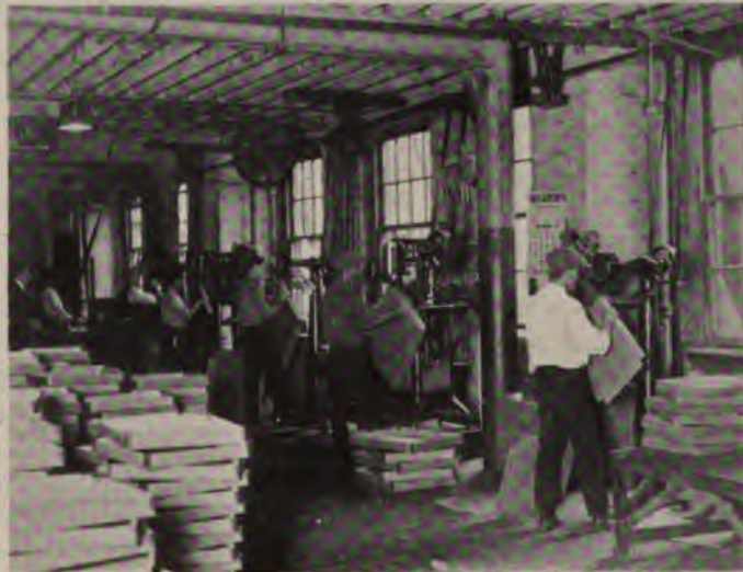
Photograph by The New York Edison Company
