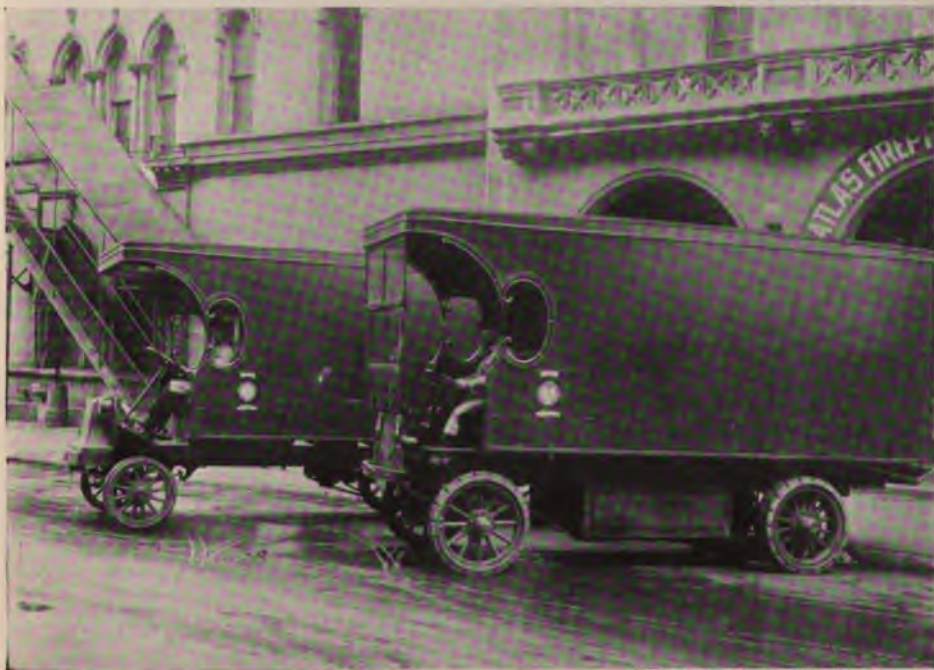
Photograph by The New York Edison Company
