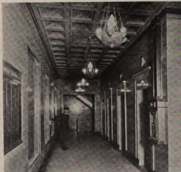
Photograph by The New York Edison Company Four Electric Elevators Provide Rapid Service for the Building Tenants
