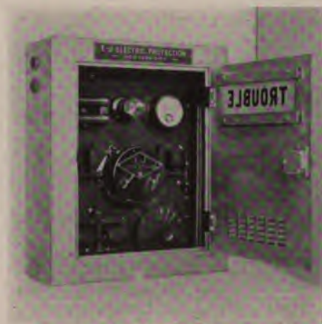
Photograph by The New York Edison Company
