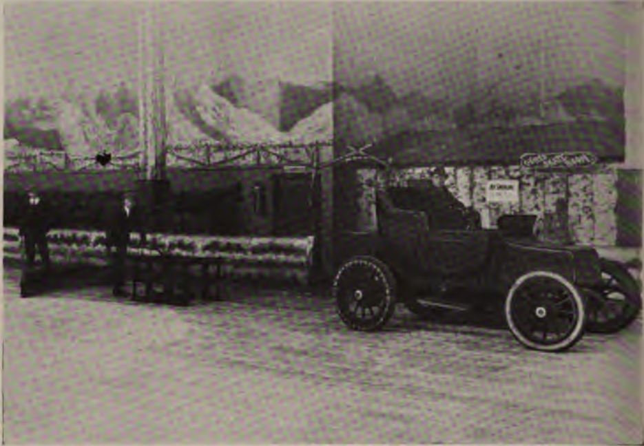
Photograph by The New York Edison Company
