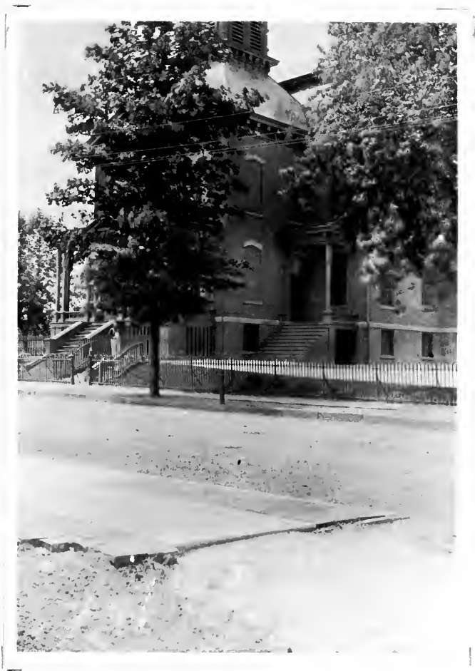
Old School, No. 1. Showing old front and iron fence. Note old hitching post in front. (Figure is janitor John Olmenhiser)
