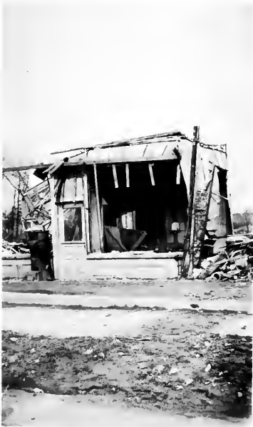
Academy Dist. Sch. in process of demolition.
