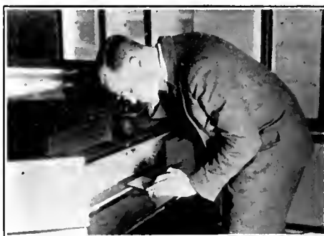
A Device That Measures the Bending of a Steel Rail under the Pressure of a Finger.
