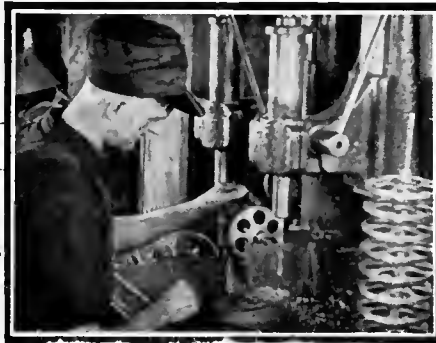
Balancing Spindle Driving Gear
