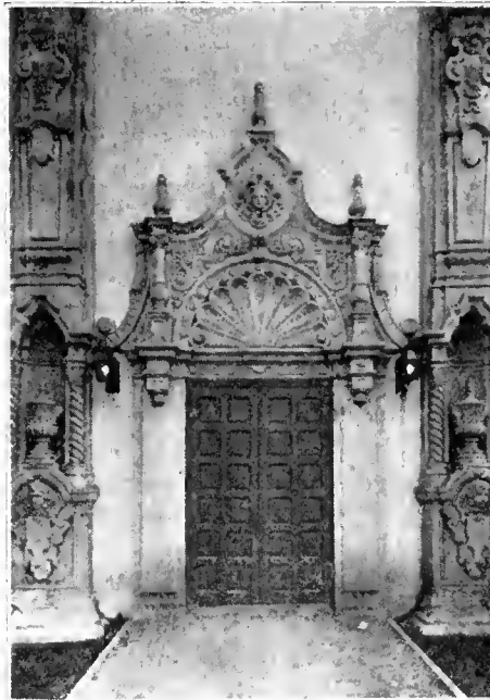
Side entrance, United States Cinema Building, International Exposition at Seville.
