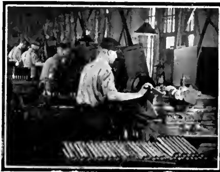
Machining Crankshafts
