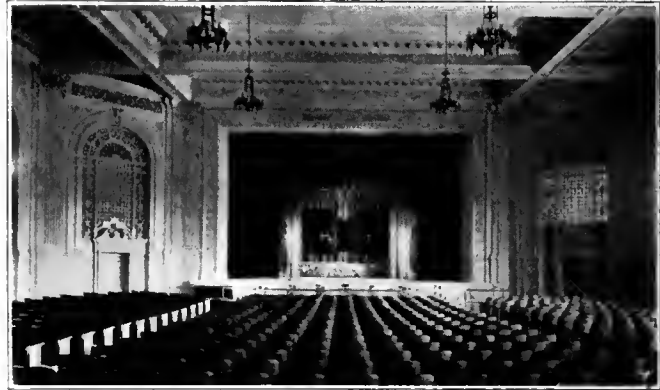
Screen Is Raised To Show Horn Used in Assembly Hall
