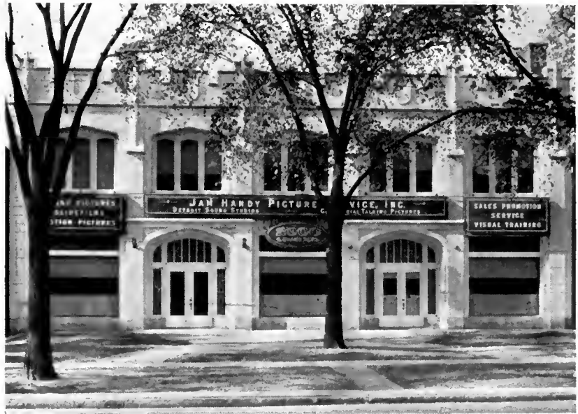
The Jam Handy Studio in Detroit, from a photograph made about 1929. A remodelled church, with offices in front and the stages and workshops in the rear. Over and over through the centuries the drama has been fostered by the church, but probably never more literally than this.
