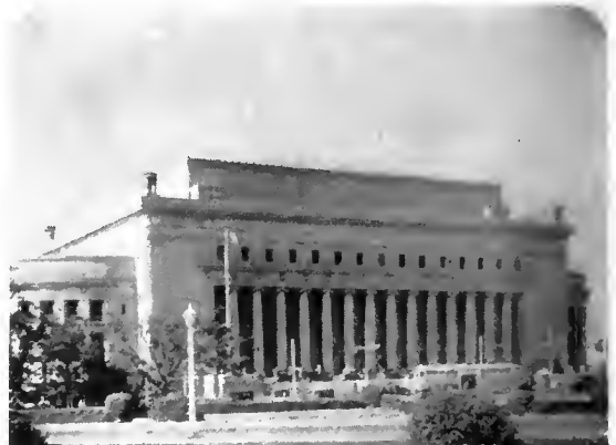
Bureau of Posts Building, Philippines
