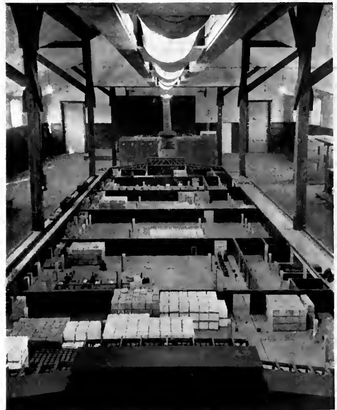
A 35x14 foot roofless model of a standard Army warehouse, built on a scale of one-half inch to the foot, gives the soldier student a realistic conception of warehouse layout without actually going to see one.
