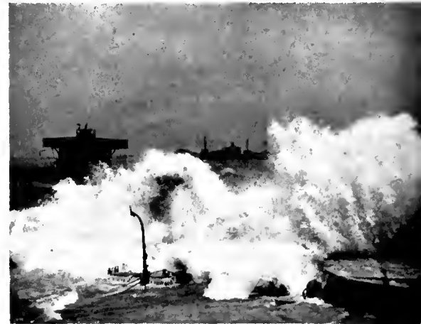
Strategic sinking of 23 freighters created breakwater behind which the Allies unloaded troops and supplies in storm that ripped Normandy beach.
