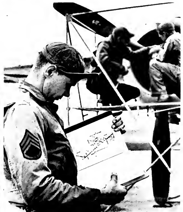
(Below) An Air Forces mechanic consults photographic "exploded views" contained in his service manual before tackling a maintenance job. These illustrations, which show photographically the exact relationship of parts in vital war equipment, are used in instruction manuals of the armed forces to eliminate guesswork and "tinkering". Using this type of visual aid, Jack Butler, 11-year-old Chicago "Whiz Kid", assembled an aircraft carburetor in less than two hours in a test conducted by Bendix Aviation Corporation.
