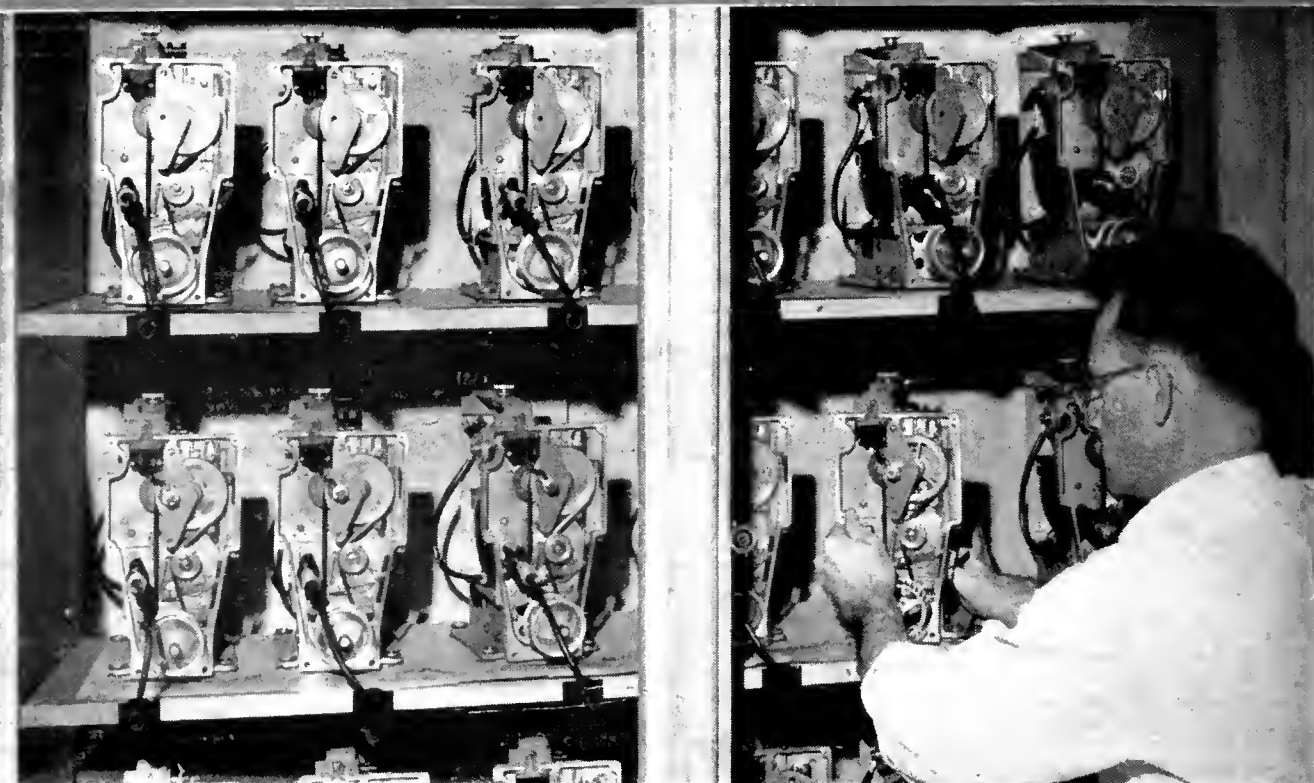
Operation of projector mechanisms in "run-in" cabinet is one of many quality controls that assures long life of Victor projectors.
