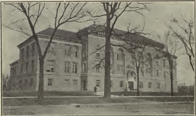
EASTERN HIGH SCHOOL, 1901 Boulevard and Mack Avenue
