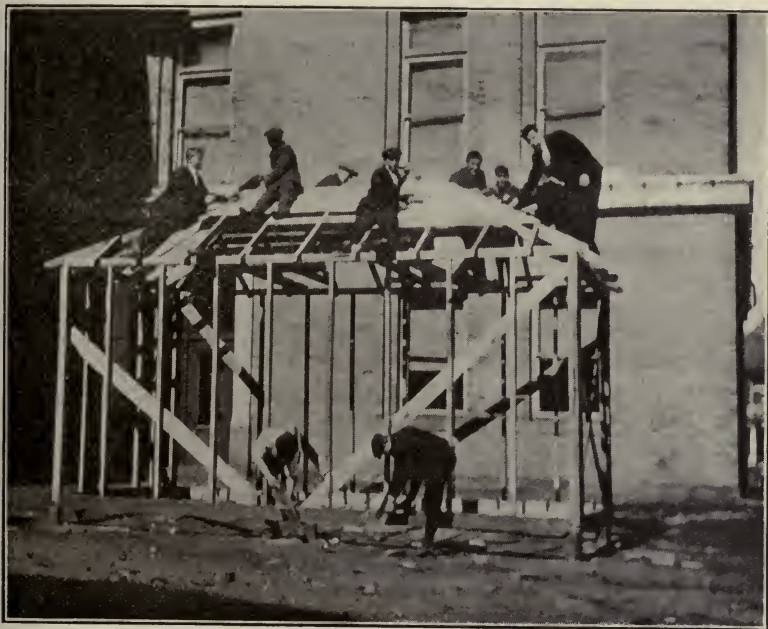
BOYS BUILDING GARAGE.
