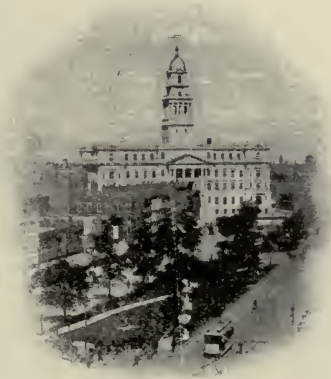
COUNTY BUILDING Cadillac Square
