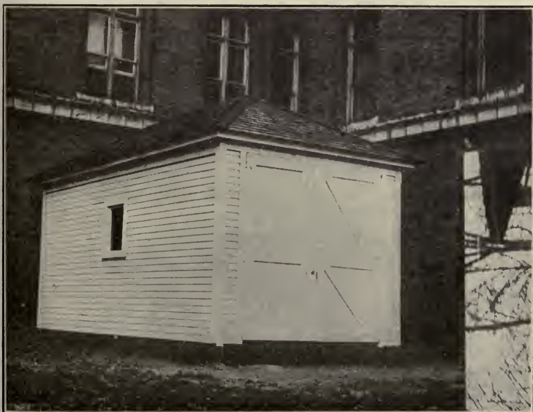
GARAGE WHEN COMPLETED.
