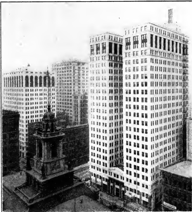
Penobscot Building Ford Building Dime Bank Building City Hall SAME AREA IN 1916
