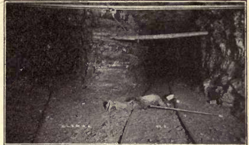
Drill Struck Wire. Miner Thrown to Ground
