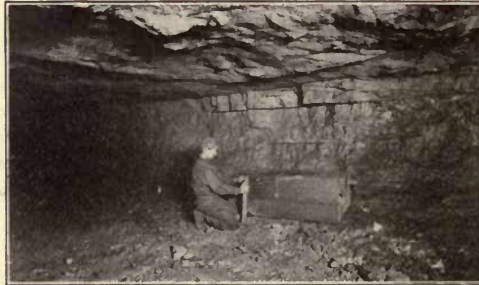
Preparing Cartridge With Lamp at a Safe Distance
