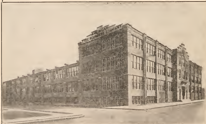
Central Plant, Jersey City, N. J.
