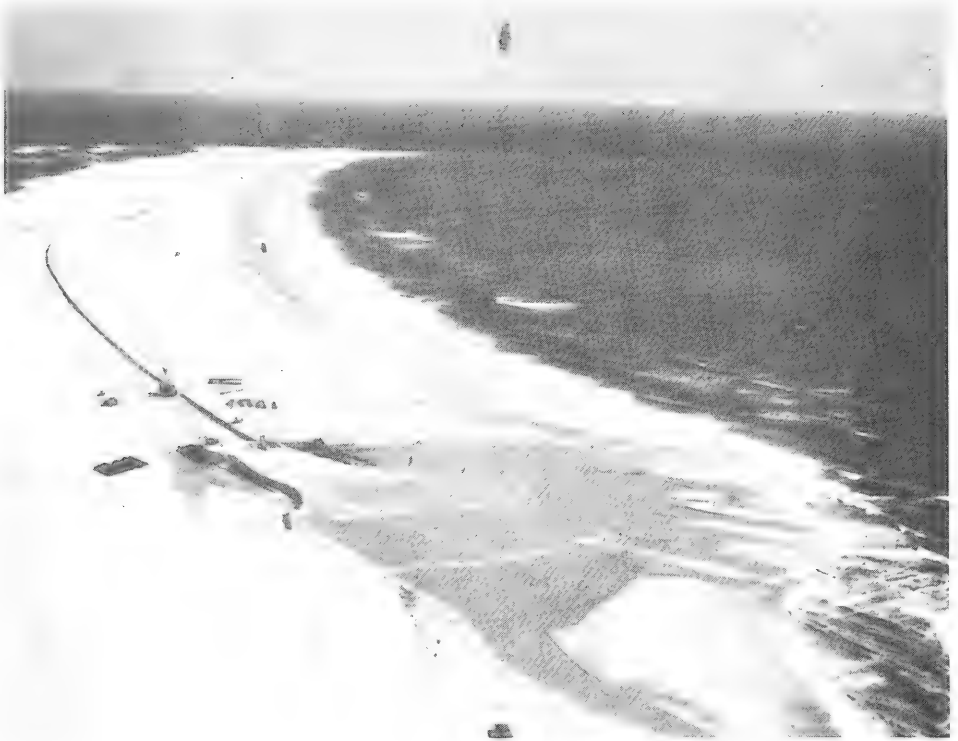
Figure 1. Beach nourishment operation, Mayport, Florida (courtesy of U.S. Army Engineer District, Jacksonville).
