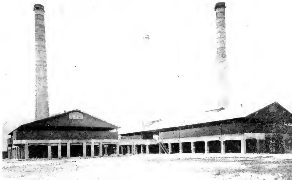
FIGURE 31. Garbage and rubbish incinerators at Kyoto.
