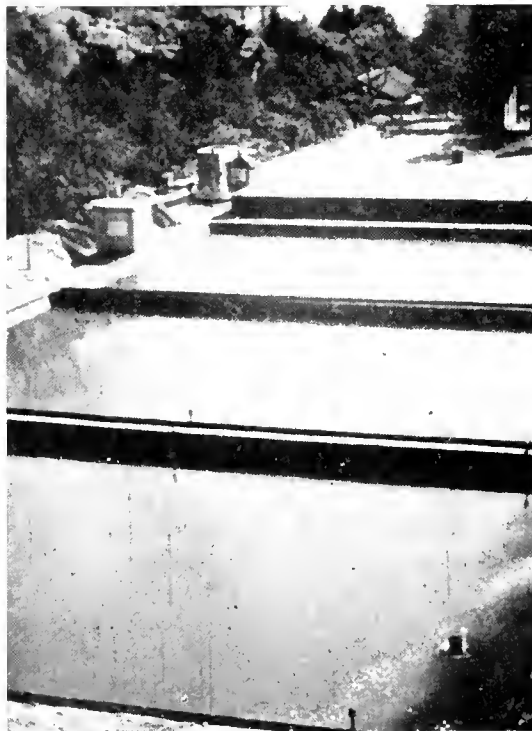
FIGURE 15. Slow sand filter in operation.
