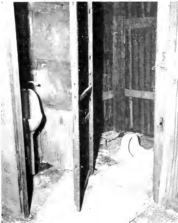
FIGURE 21. Japanese toilet (Benjo) consisting of urinal and "squat" bowl mounted over a pit, housed in temporary building. Tokyo bombed area.
