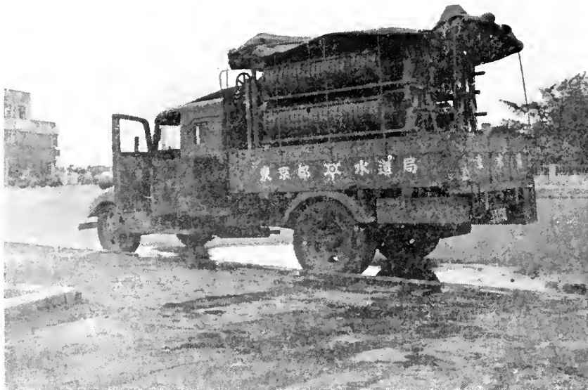
FIGURE 16. Portable emergency filter for supplying drinking water.
