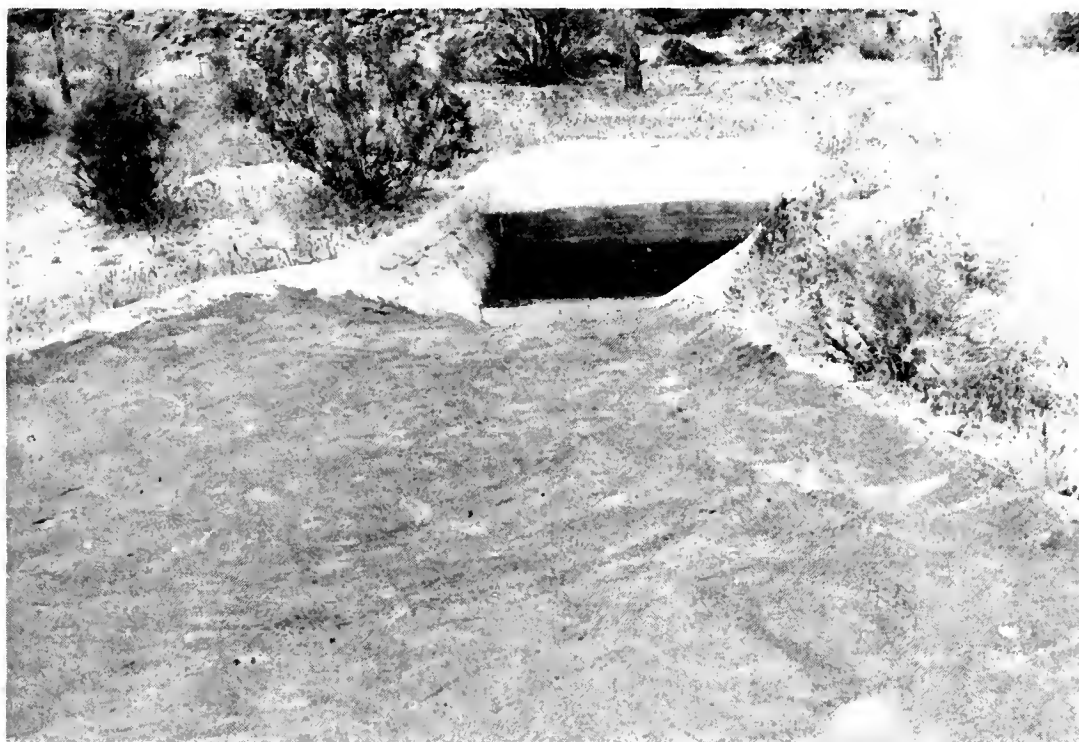
Figure 12. Concrete open-basin type water catchment.
