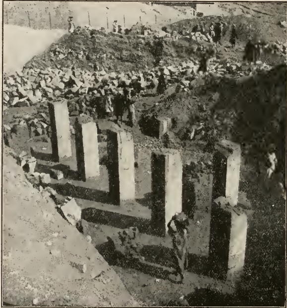
EXCAVATION OF THE NORTH LOWER COLONNADE OF THE XIth DYNASTY TEMPLE, DÊR EL-BAHARI, 1904.
