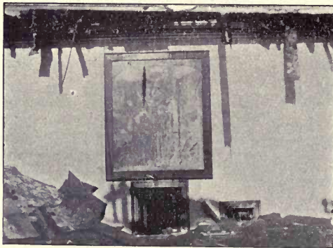
COURT ROOM AFTER THE FIRE.
