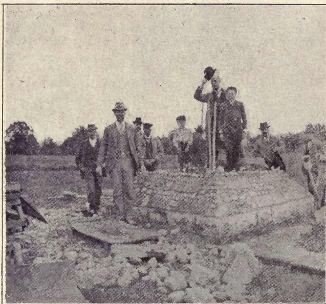
Judge Ermatinger and Dr. Bartlett, Treasurer, placing Records and Coins in Cairn Contractor G. A. Ponsford in foreground
