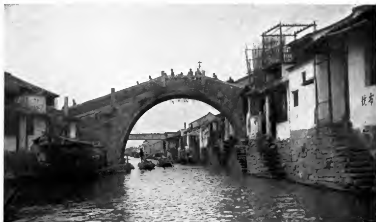
SOUTH HORSE ROAD BRIDGE, OVER THE T'SI MEN CANAL, SOOCHOW.
