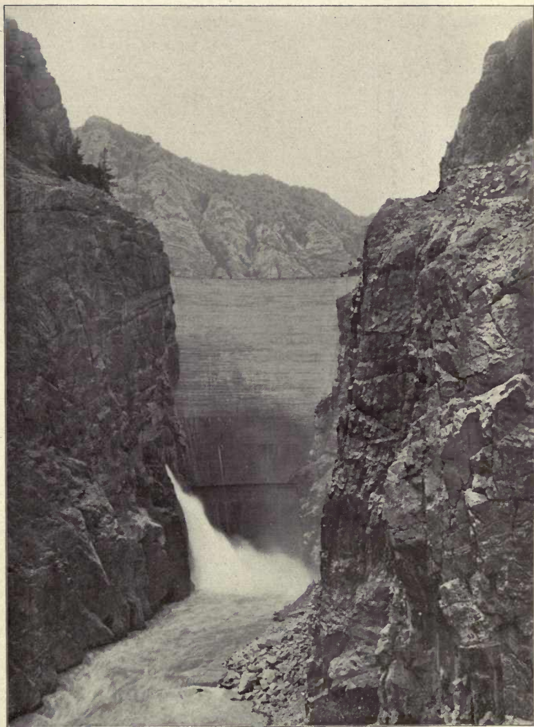
PL. VIII. Shoshone dam, (highest in the world, 327 feet high) on Shoshone River east of Yellowstone Park, Wyo., for holding flood waters.
