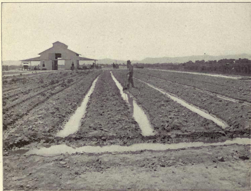
PL. VB. Methods of distributing irrigation water to the desert lands.
