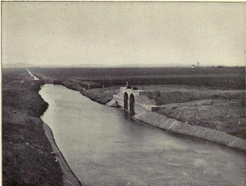
PL. VIA. Distributing canal and structures on North Platte project, Nebraska.
