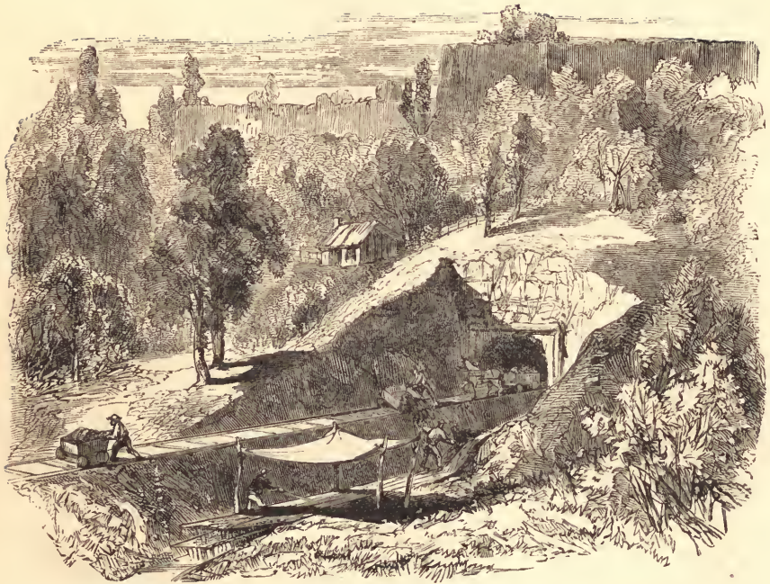
TUNNELLING AT TABLE MOUNTAIN, CALIFORNIA.
