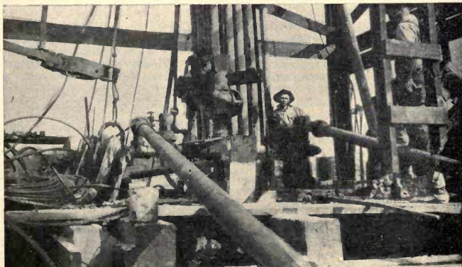
Plate II—Bailing Down to Bring in Well. Connections Made for Flowing Well.
