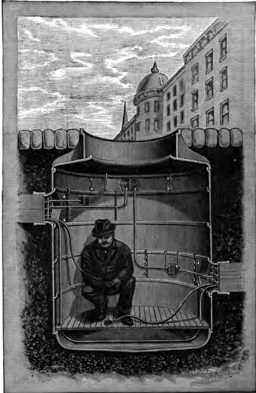
Manhole of the Johnstone Conduit System.
