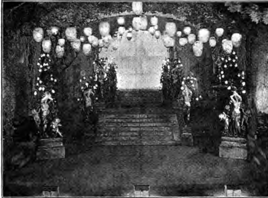
Electric Lighting at the Tyne Theatre—Andrews' Concentric Wiring.
