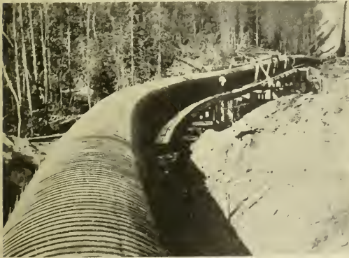
Fig. 6—66" Wood Stave Pipe Syphon, Kamloops Power Plant.
