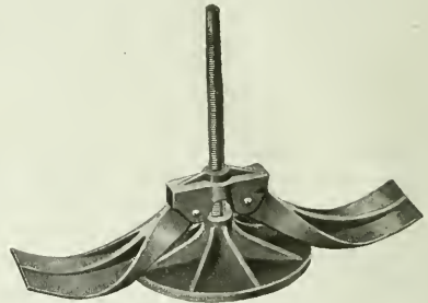
"Faultless" pole guy anchor.
