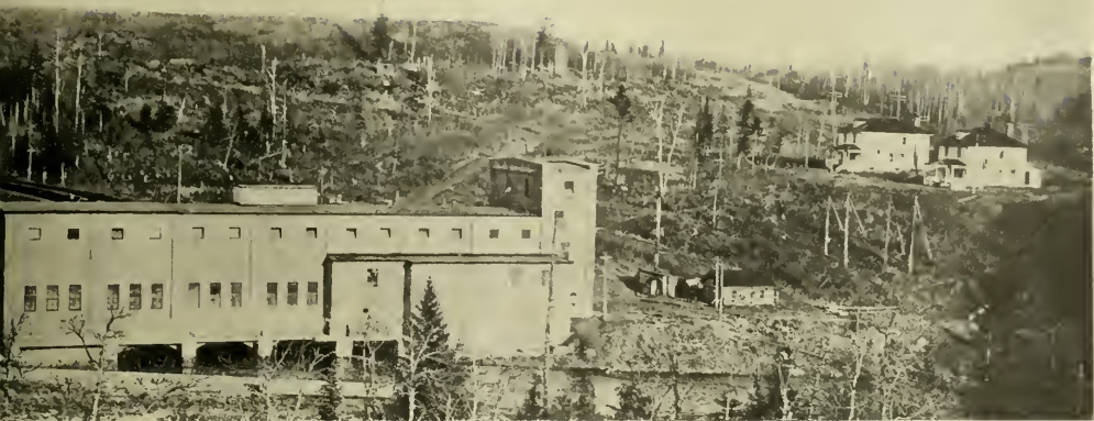
cs, Reinforced Concrete Power House and Tail Race—Kaministiquia River in Foreground and Transmission Line to the Right.
