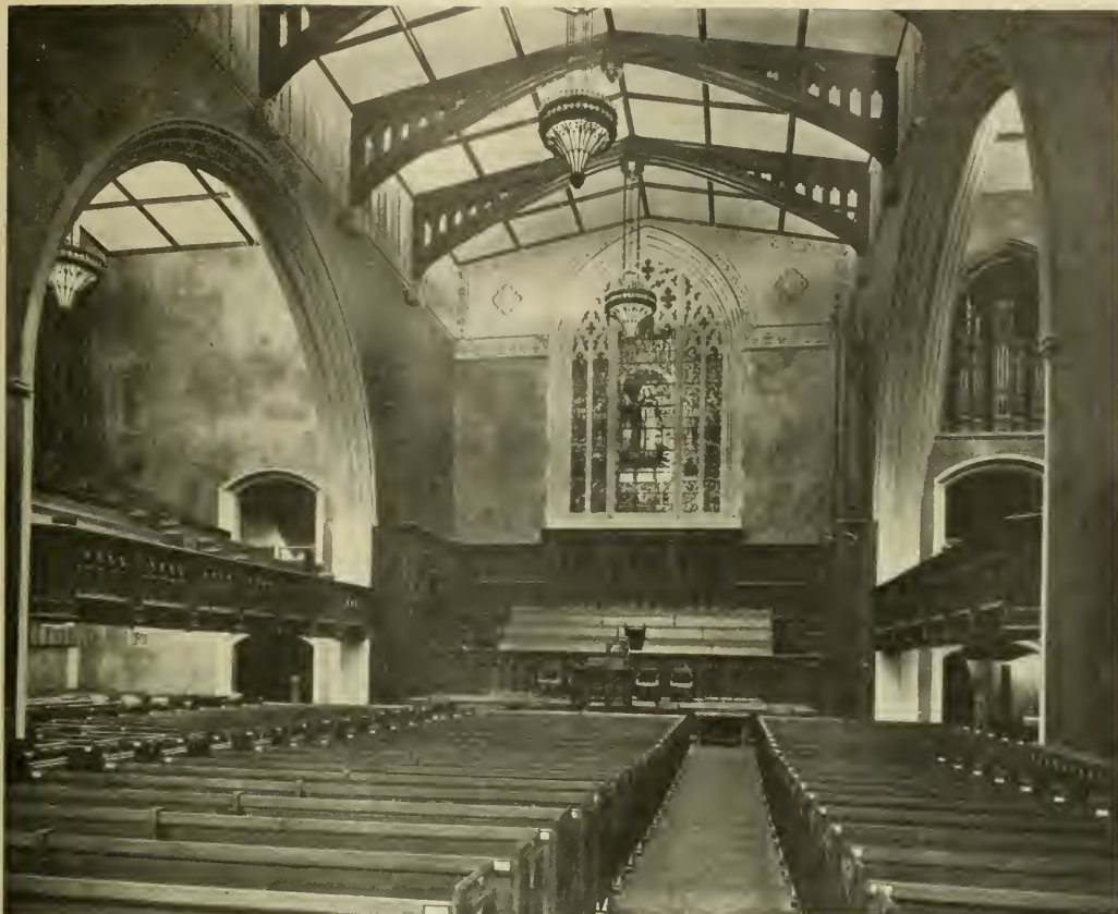
Church lighting from concealed sources—Timothy Eaton Memorial Church, Toronto.
