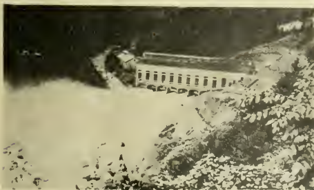
Relief valves of 6-8000 h.p. wheels discharging under head of 1500 ft.
