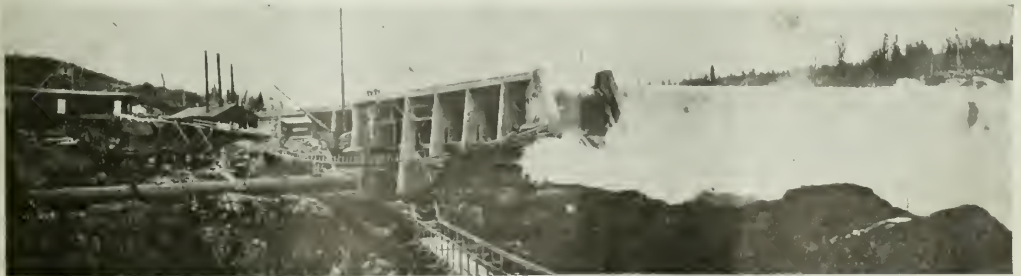
Down stream side Ambursen dam, showing penstock, bulkhead, log sluice and spillway.
