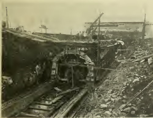
First completed section of aqueduct—Buggies used for conveying concrete from the mixers on pouring platform—Forebay in background.
