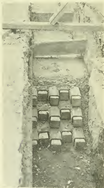
15 duct run showing concrete encasement.
