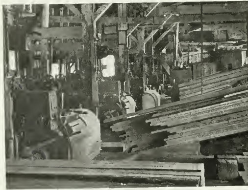
View of Electrically Driven Planing Mill
