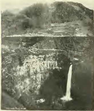
First Necaxa Falls, showing temporary plant.
