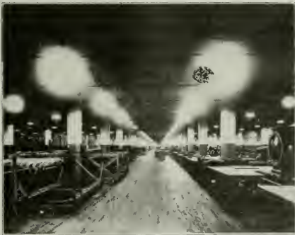
From this photograph the results of a system of general illumination are shown. Room 1,000 feet long, 66 feet wide. Shallow bowl type reflectors 10 feet high, 11 feet 6 inches apart. The intensity is high and uniform. Note the absence of glare and shadows. Photo taken at night by the illumination from the lamps and reflectors only and not retouched.
