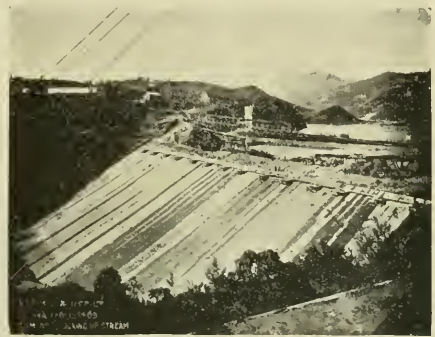
Necaxa dam, lower rockfilled toe with masonry face.
