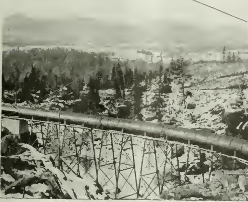
Penstock crossing gorge on steel trestle.
