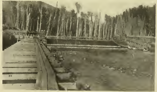
Fig. 4—Intake Dam, Hydro Plant, Kamloops, B. C.
