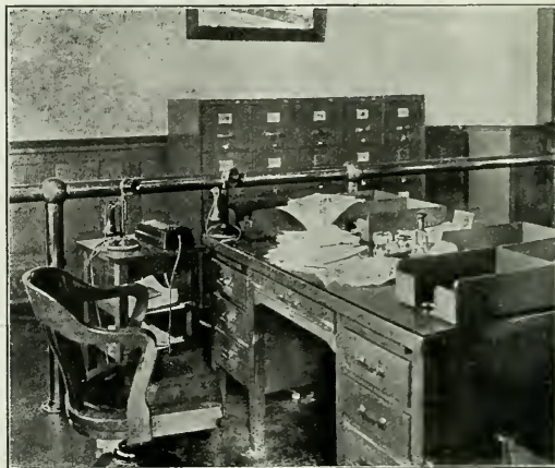
Inter communicating Telephone System in Wrigley Factory.
