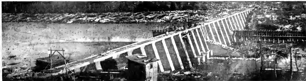
Hollow Concrete Dam at Outlet of Lake St. Francis.
