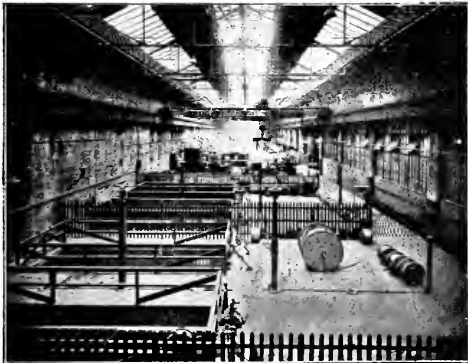
High Tension Testing Department
