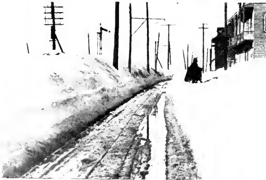
Snow several feet high on both sides of the tracks.
