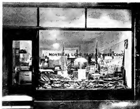
Fig. 6 — District Branch on St. Denis Street
