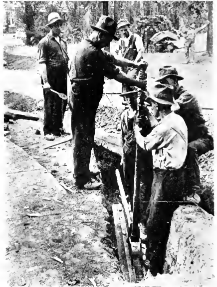
Fig. 3—Forcing pipes under the Roadway
