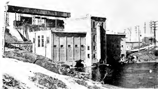
Soulanges Generating Plant, Montreal L. H. & P. Consolidated
