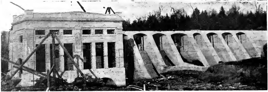
Weedon Power Plant, Sherbrooke Municipal System.
