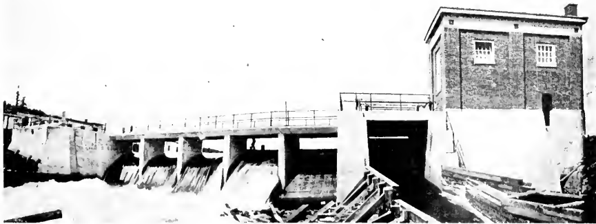
View of the Kipawa Plant of the Riordan Pulp & Paper Company
