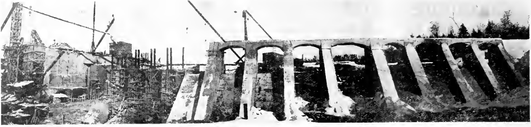
Panoramic view of hydro-electric plant at Weedon, P.Q., under construction.
