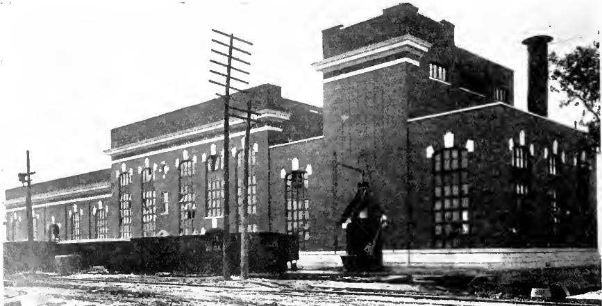
Montreal Public Service Corporation Terminal Station, Montreal.
