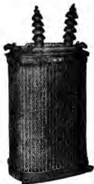
Single Phase POWER TRANSFORMER
