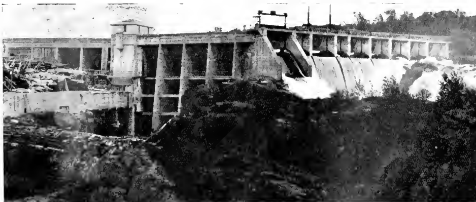
Dam of Laurentian Power Co. on St. Anne River.
