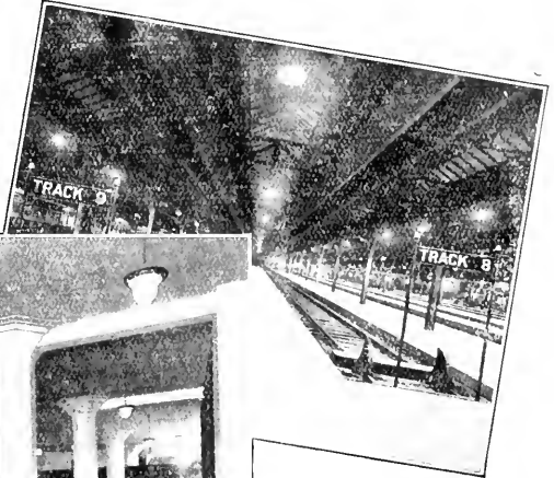
Lighting Installation in Windsor Station Montreal
