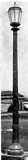
Fig. 1: Lighting Standards to be installed on the Humber Boulevard. They will be mounted 100 feet apart and carry 1000 c. p., 20 ampere, series lamps. Each standard will be equipped with its own transformer housed in the base.
