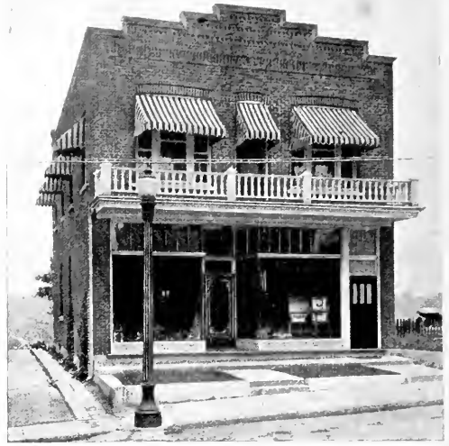
Drummondville Office and Store, Southern Canada Power Co.
