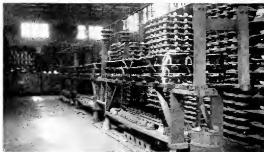
Fig. 3. A Rack of Insulators Ready for Test.
