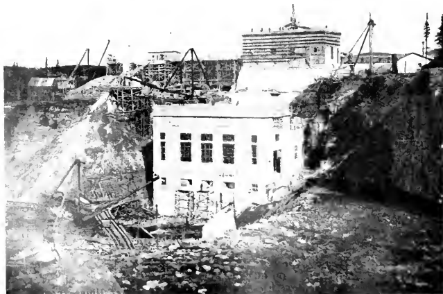
Price Bros. power house at Chute aux Galets—One of the most modern plants on the continent.
