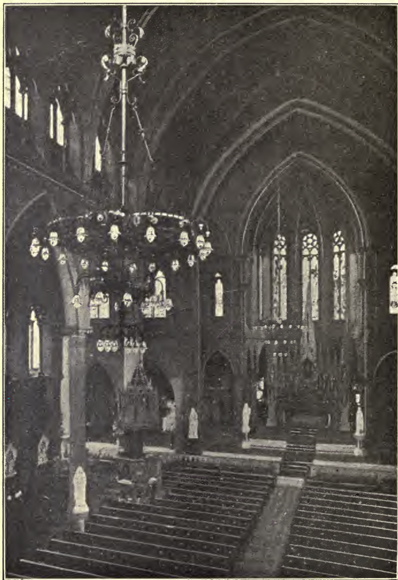
FIG. 7'26.—Lighting Installation of the Holy Name Church, Manchester.
