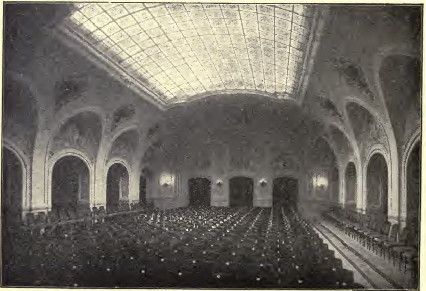
FIG. 7·24.—Arc Lamps above a Glass Ceiling.
