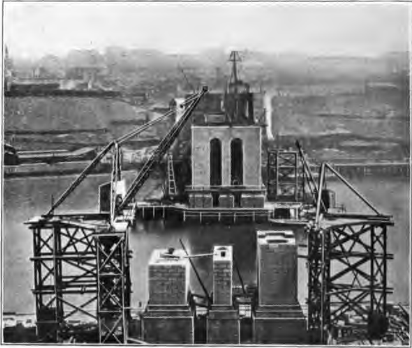
Fig. 332.—Derrick Cranes Erecting Piers.
