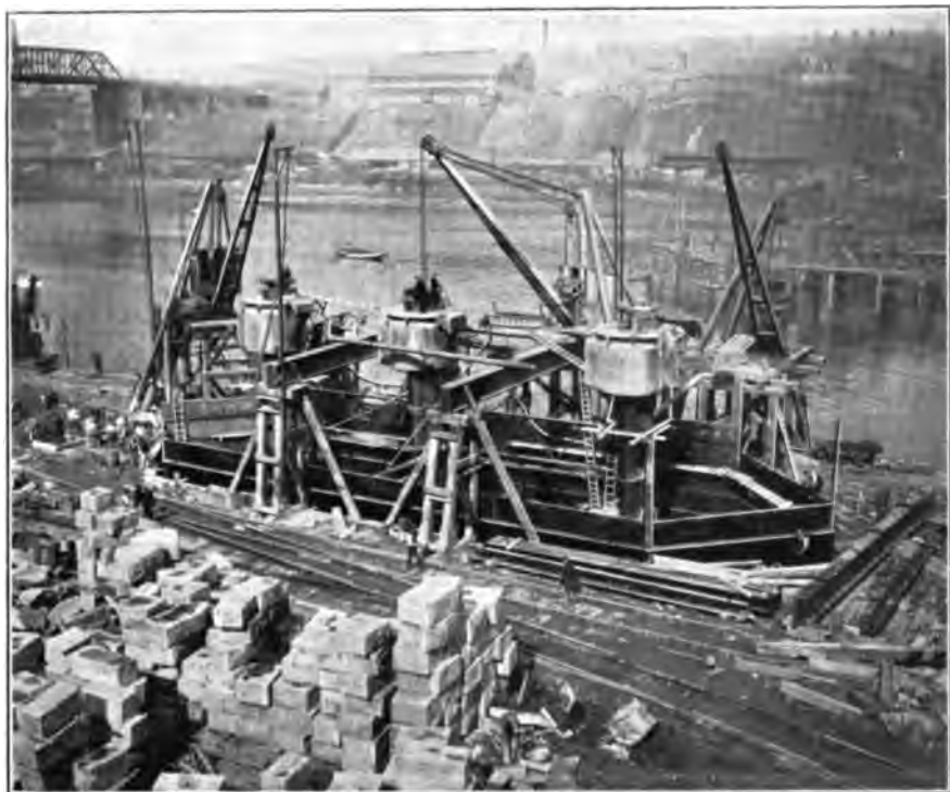
Fig. 330.—Derrick Cranes on Caisson.
